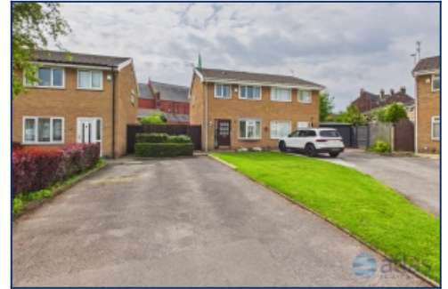
Front Elevation Of Property & Driveway
