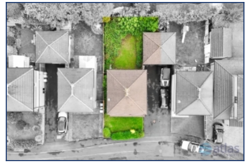
Aerial Front Boundary
