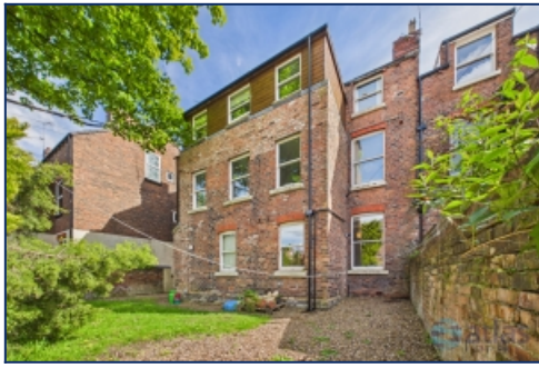
Rear Elevation Of Property
