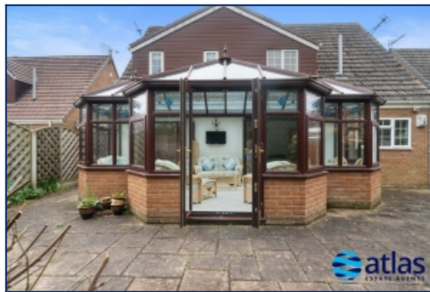
Rear Elevation Of Property
