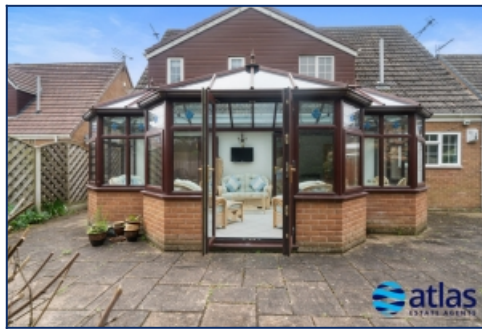
Rear Elevation Of Property
