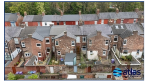
Aerial View Rear
