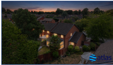
Aerial Rear Elevation (night Shot)
