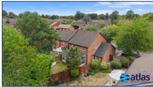
Aerial Rear Elevation
