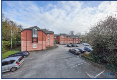
Rear Elevation Of Property
