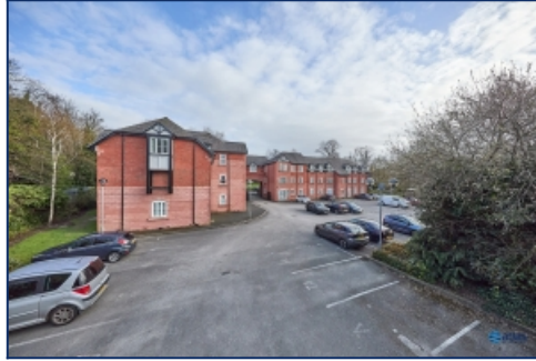
Rear Elevation Of Property
