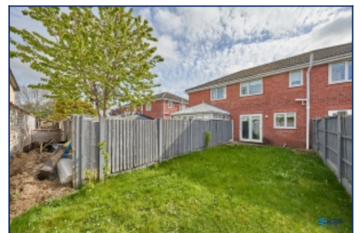
Rear Elevation Of Property
