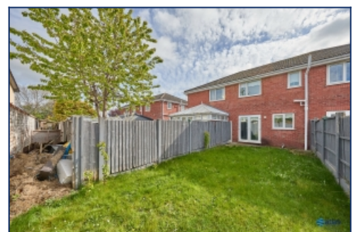
Rear Elevation Of Property
