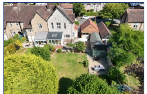
Aerial Rear Elevation
