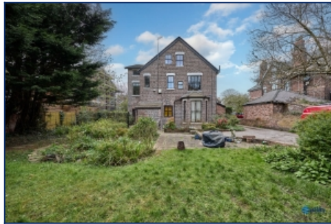
Rear Elevation Of Property
