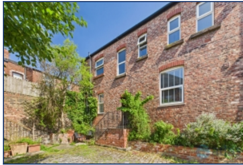
Rear Elevation Of Property
