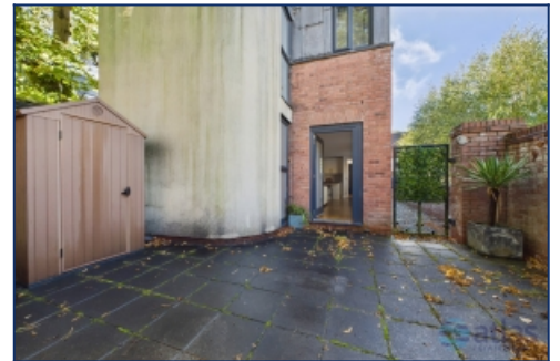
Rear Elevation & Rear Yard
