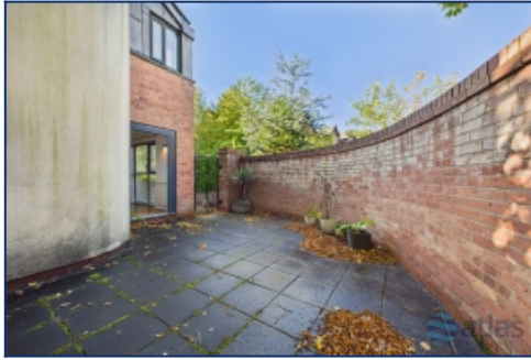
Rear Elevation & Rear Yard
