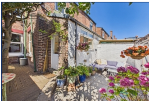
Rear Elevation & Rear Yard
