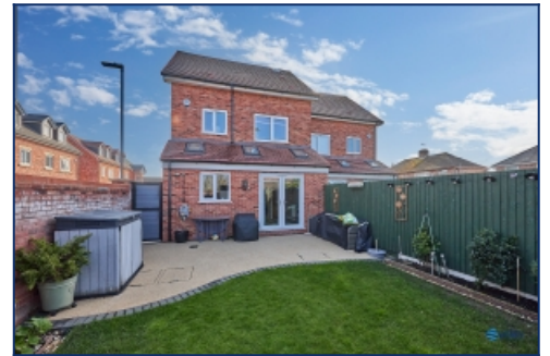
Rear Elevation Of Property
