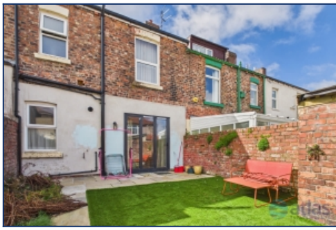
Rear Elevation Of Property
