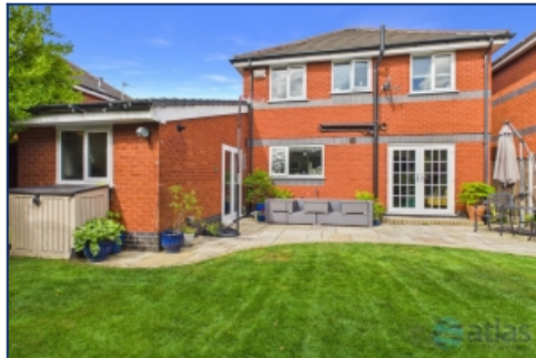
Rear Elevation Of Property
