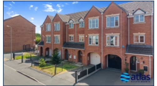
Aerial Front Elevation
