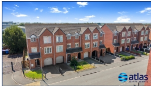
Aerial Front Elevation
