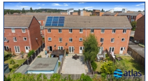
Aerial Rear Elevation
