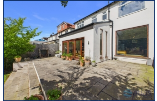
Rear Elevation Of Property
