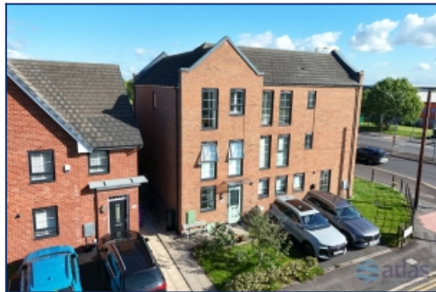
Aerial Front Elevation
