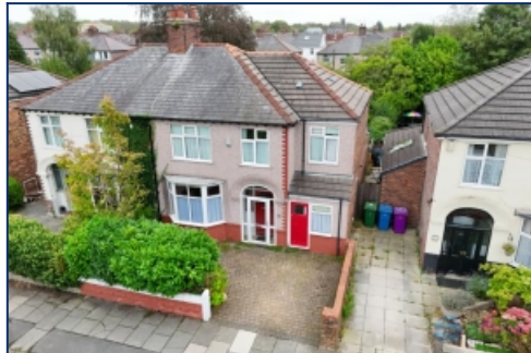
Aerial Front Elevation
