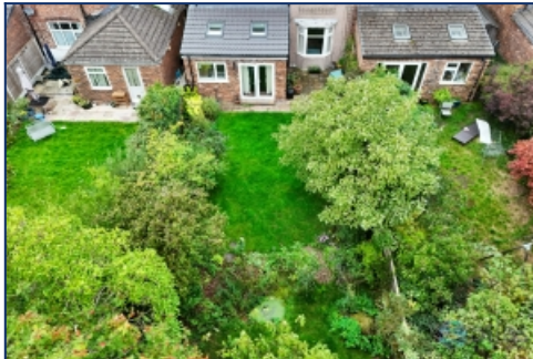
Aerial Rear Elevation & Garden
