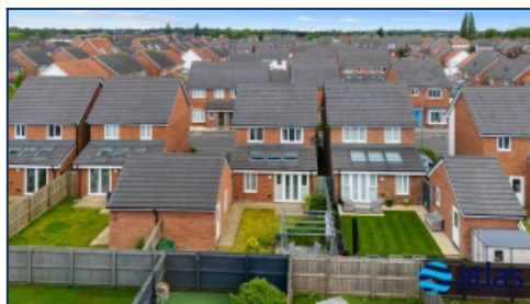
Rear Elevation Of Property
