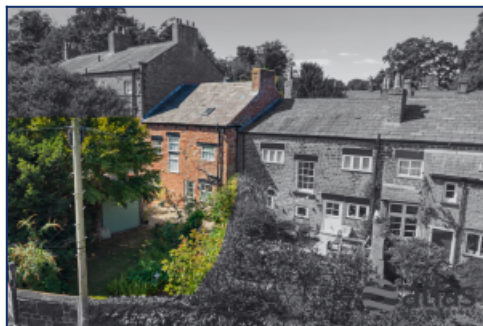
Rear Elevation Aerial View Boundary
