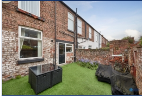
Rear Elevation Of Property
