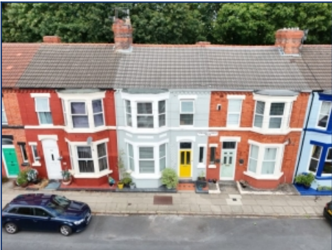
Aerial Front Elevation
