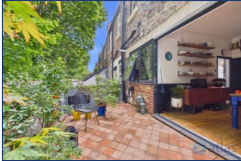
Rear Elevation & Rear Yard
