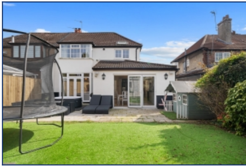
Rear Elevation Of Property
