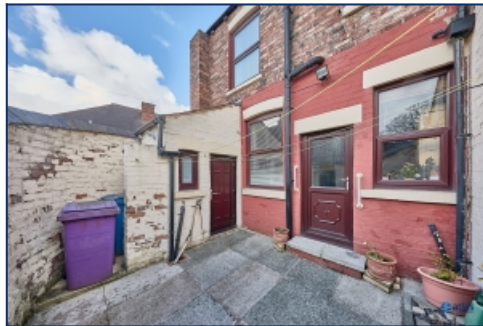
Rear Elevation Of Property
