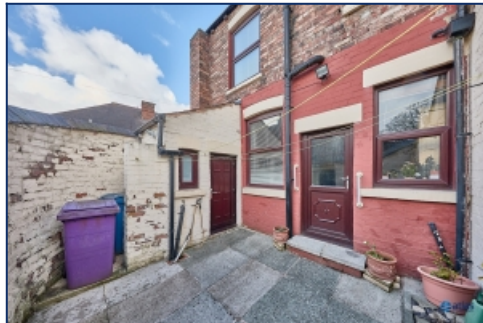
Rear Elevation Of Property
