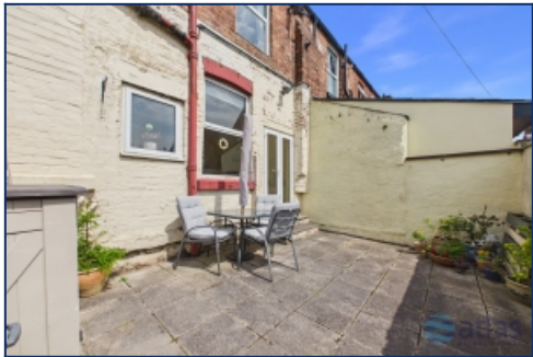
Rear Elevation Of Property
