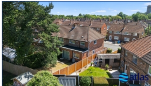
Rear Elevation Of Property
