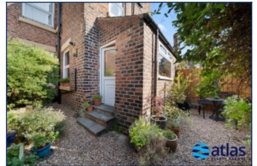
Rear Elevation & Rear Yard
