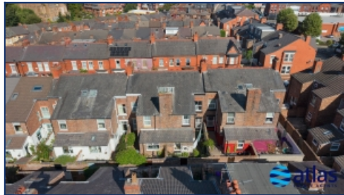
Aerial Rear Elevation
