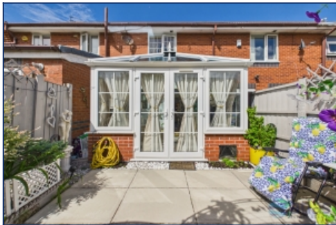
Rear Elevation Of Property
