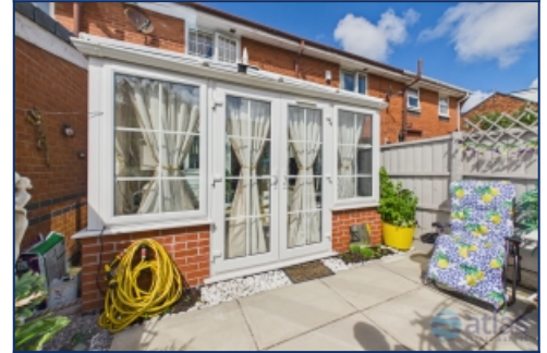
Rear Elevation Of Property
