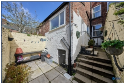
Rear Elevation Of Property
