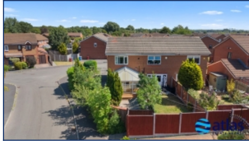
Aerial Rear Elevation
