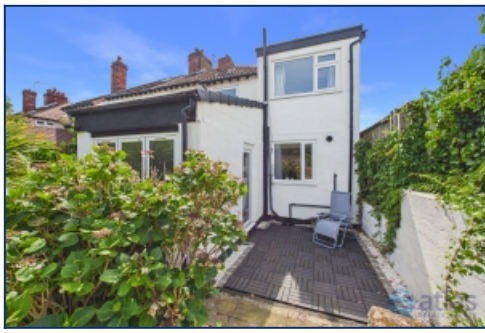
Rear Elevation Of Property
