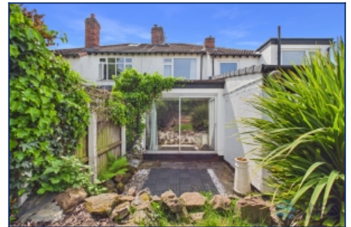
Rear Elevation Of Property
