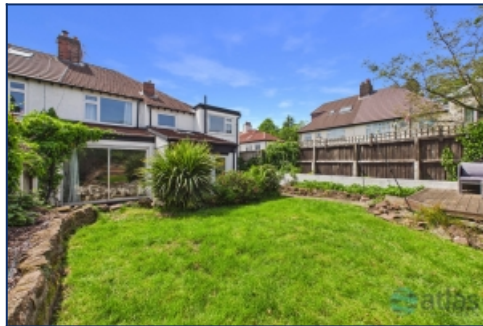
Rear Elevation Of Property
