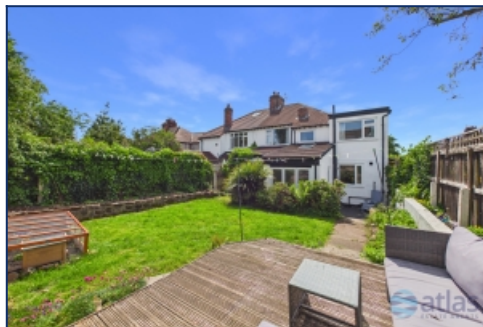
Rear Elevation Of Property
