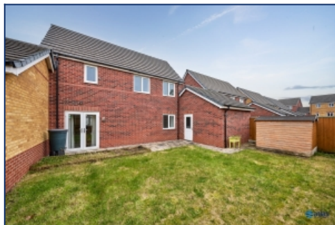
Rear Elevation Of Property
