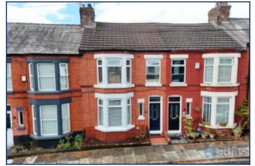
Aerial Front Elevation
