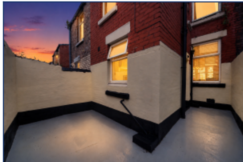
Rear Elevation Of Property & Outdoor Space (night Shot)
