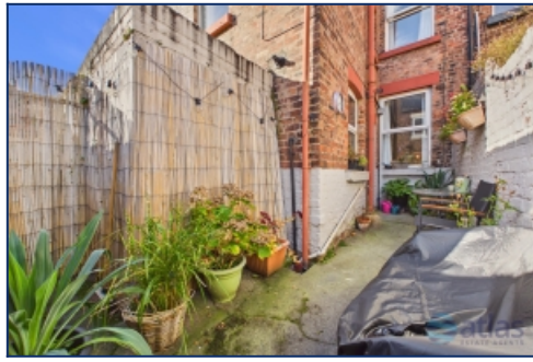
Rear Elevation & Yard
