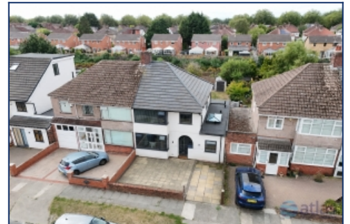
Aerial Front Elevation
