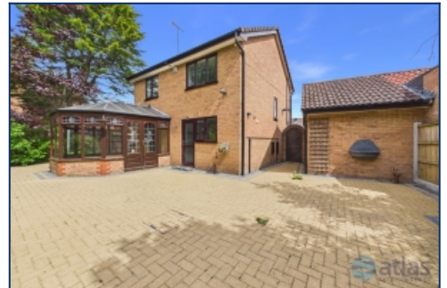
Rear Elevation Of Property
