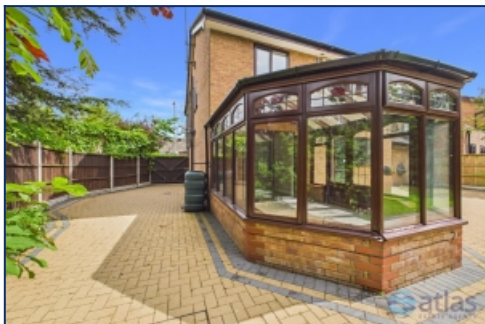
Rear Elevation Of Property
