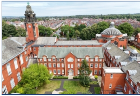
Aerial View Of Building
