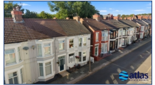
Aerial Front Elevation
