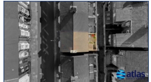
Aerial View Boundary
