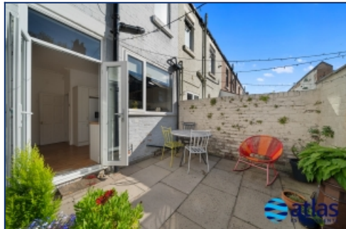
Rear Elevation & Rear Yard
