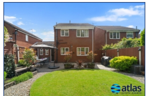
Rear Elevation Of Property
