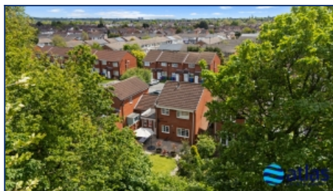
Aerial Rear Elevation
