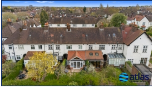
Aerial View Rear
