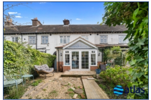
Rear Elevation Of Property
