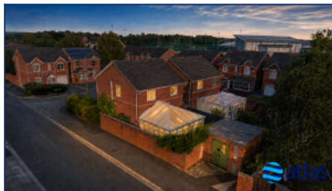
Aerial Rear Elevation (night Shot)
