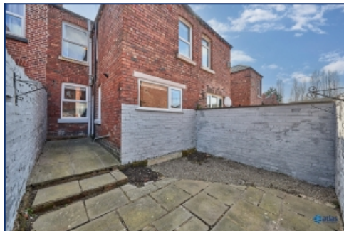
Rear Elevation Of Property
