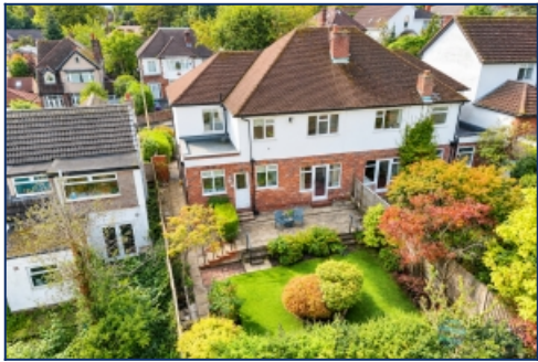
Aerial Rear Elevation
