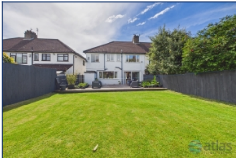
Rear Elevation Of Property
