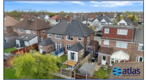
Aerial View Rear
