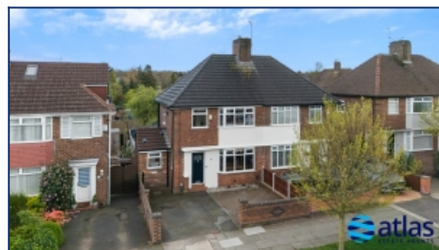
Aerial Front Elevation
