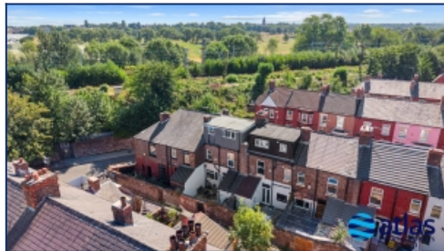
Aerial Rear Elevation
