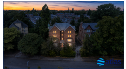
Aerial Front Elevation (night Shot)
